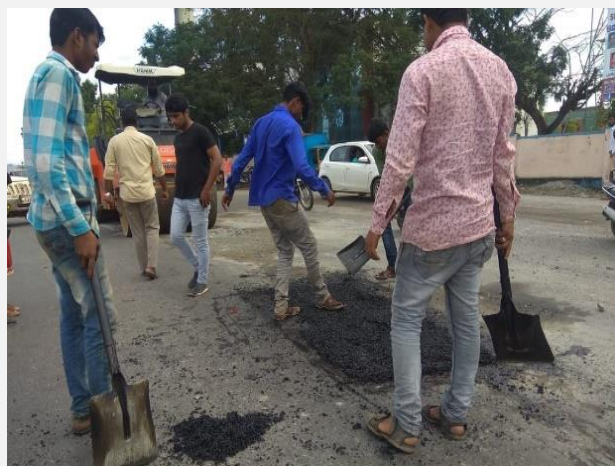
Readymade pothole mix on NH206 Road
